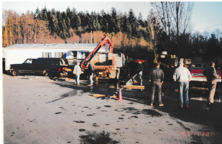
The crane ready to pull
